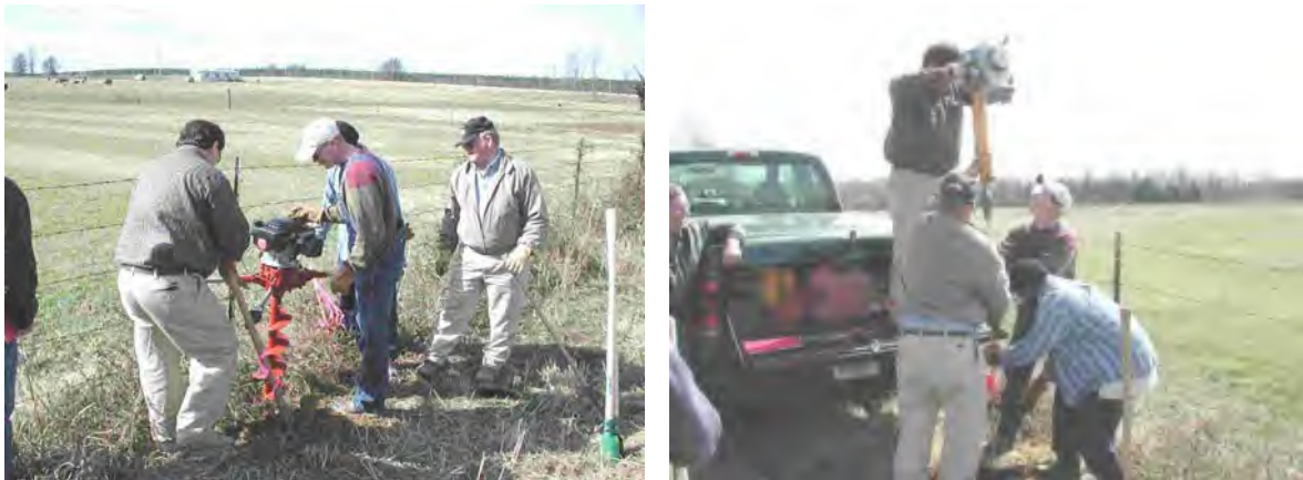
Figure 8-11. Setting deep-driven bench marks (Memphis District & 3001, Inc.)
